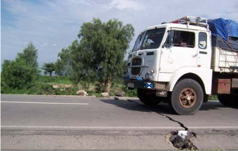
Asphalt crack
