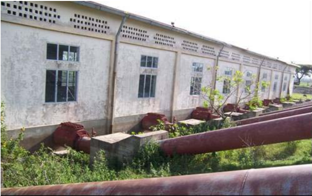
Pumping station from lake Ziway
