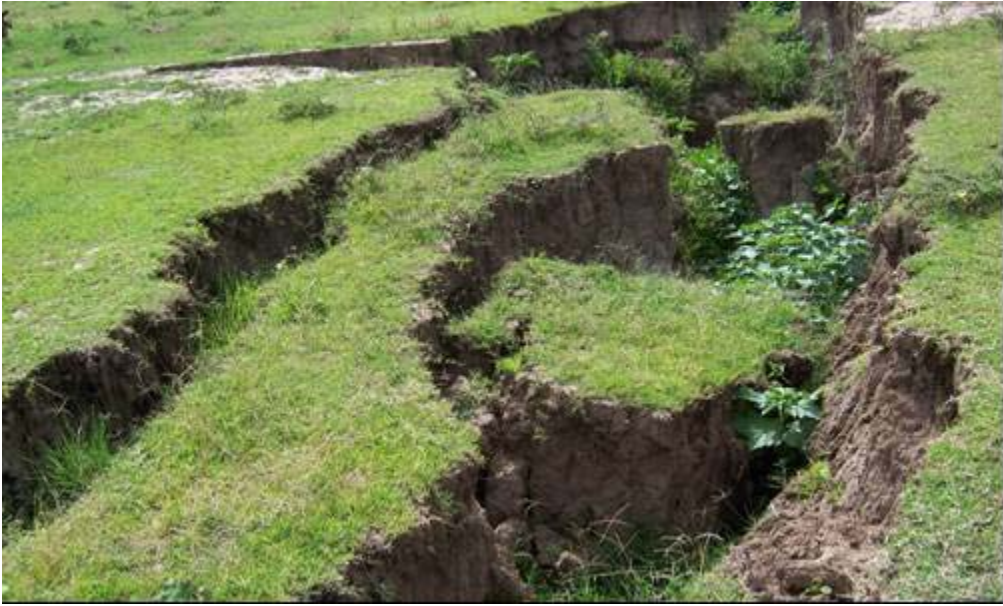
Land slide due to ground crack
