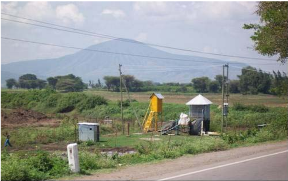
Bore hole close to Awash river
